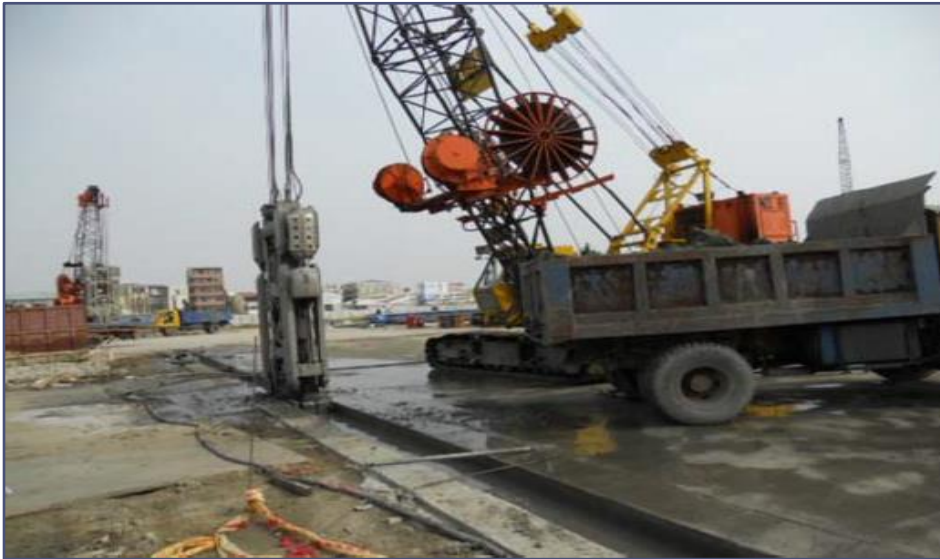
Figure G: Slurry Wall Installation (Chen, 2013)
